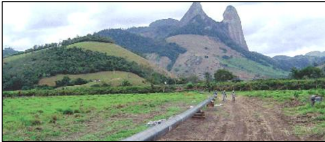
Fig. 1: Horizontal slurry carrying pipeline system, http://www.tenaris.com/en/Products/OnshoreLinePipe/Minera/SlurryPipelines.aspx
