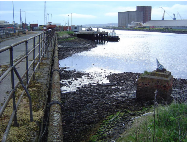
Site of storm-water outfall
