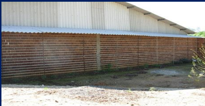
Figure 2 Porous wall (inlet)
